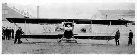
Model E-4. This is identical with JR-1-B, except for overhang. It mounts a 150 H.P. Hispano-Suiza Engine
