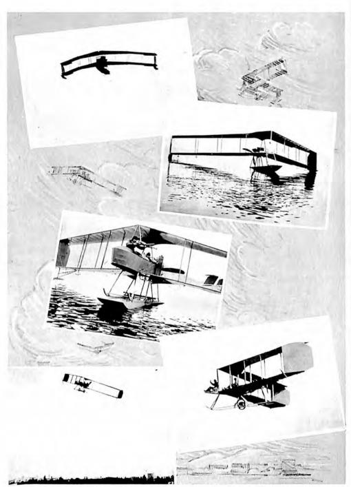
From top to bottom: 1 and 2—Burgess-Dunne Sporting Type Seaplane; 3—Burgess-Dunne Type, with Rapid Fire Gun; 4—Burgess-Dunne Land Machine, showing pilot, with locked levers, flying "handsoff"; 5—Burgess-Dunne Type Aeroplane, built for United States Signal Corps.
