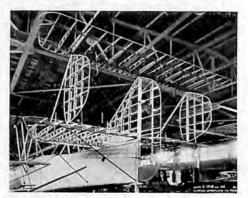
Tail Construction, Model T Flying Boat
